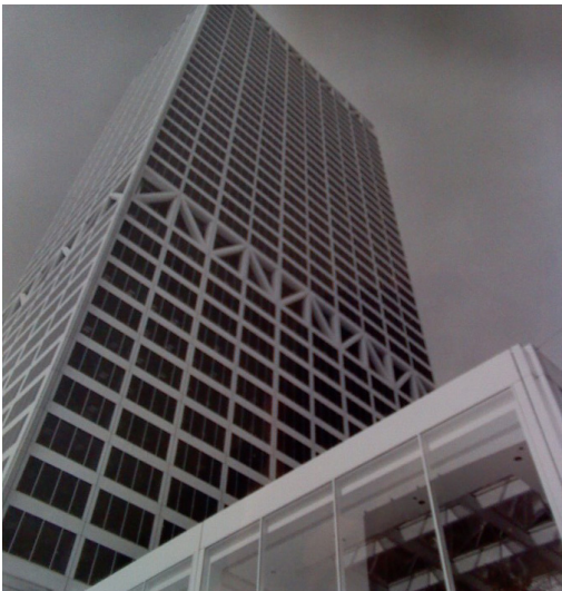
Above: original headquarters
